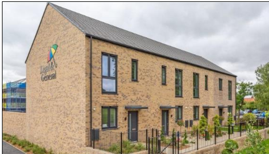
Fig.7: Applicant’s development in Selby, North Yorkshire
